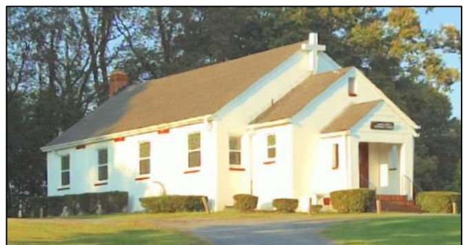
Dating to 1885, Asbury Methodist Church on Black Rock Road memorializes the Brownstown African-American community, named for one of its first landowners. Its school, nearby on Germantown Road, had been a white school until no longer needed as such. A separate residential area, Pine Top , was about a mile away off Riffle Ford Road. (2014 Microsoft Maps image)
