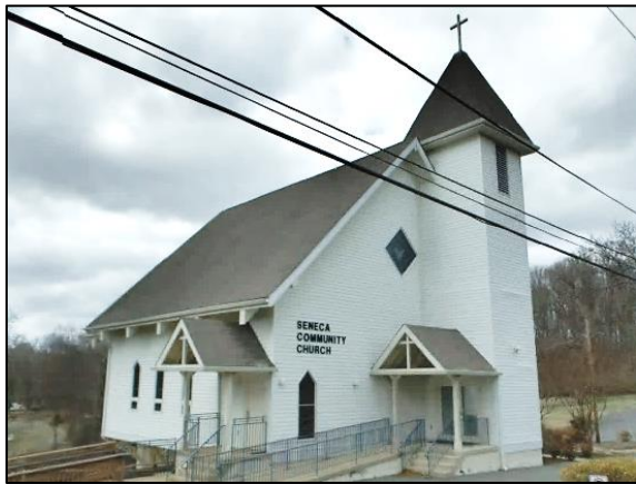
Seneca Community Church, the center of a small community on Berryville Road , was originally Potomac Grove CME (Colored Methodist Episcopal) Church on Violettes Lock Road; it relocated to this site around 1940, changed its name, and built this structure in 1999. (2022 Microsoft Maps image)
