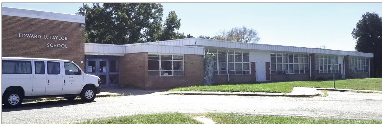
Edward U. Taylor school, located at 19501 White Ground Road, looks today much as it did when serving as the county’s only integrated mainstream elementary school beginning in 1960. (Author photo)
